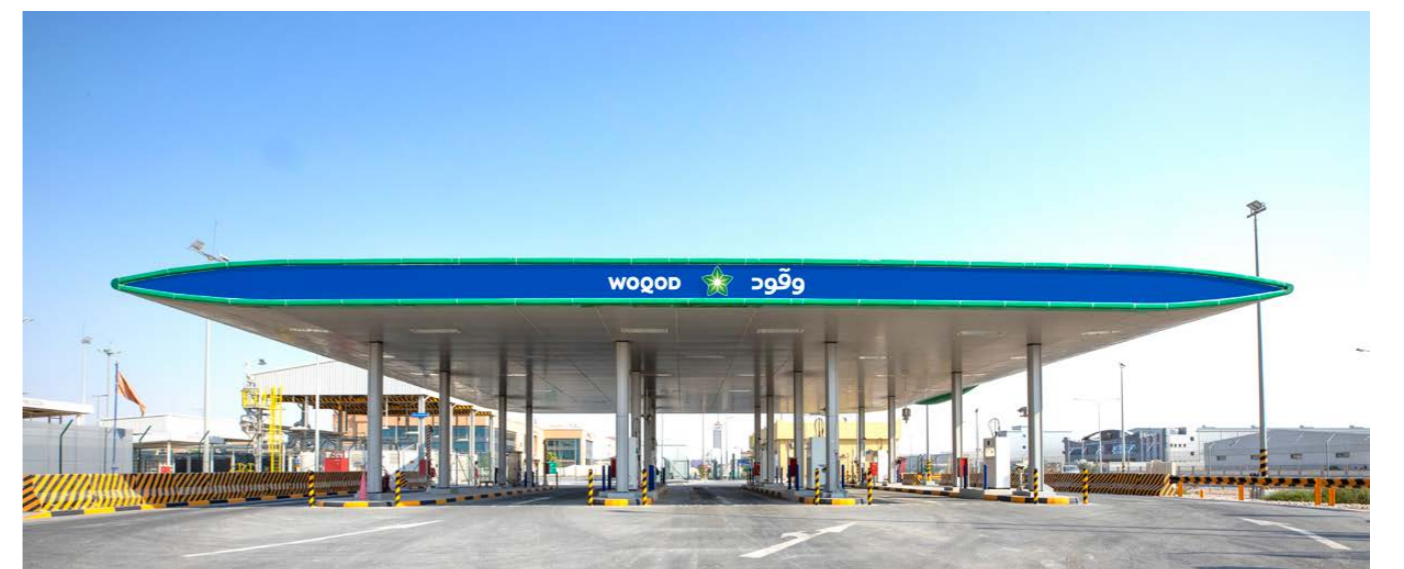
CNG fueling station at Ras Laffan
